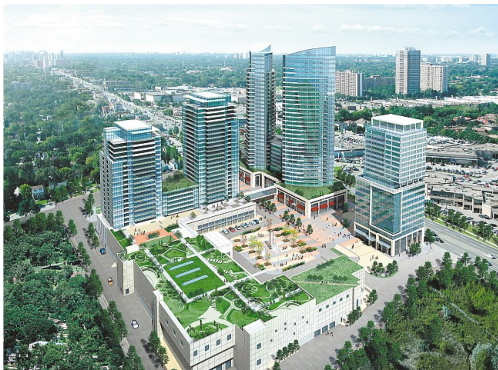
DANNY ROTH, BRANDON COMMUNICATIONS INC.
